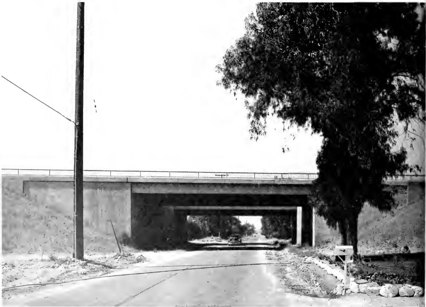
Freeway structure viewed from Monte Visto Avenue
